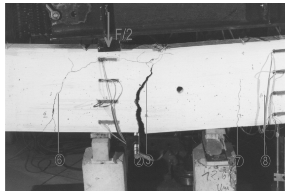
Fig. 4 Close-up around the crack that caused the failure for beam I.
